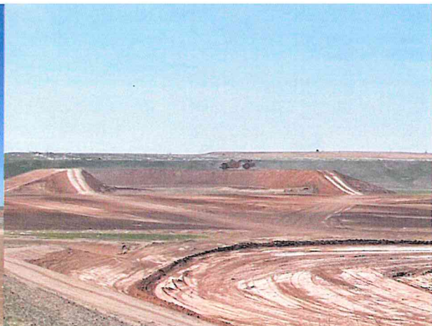
Scrapers hauling dirt to the berm
