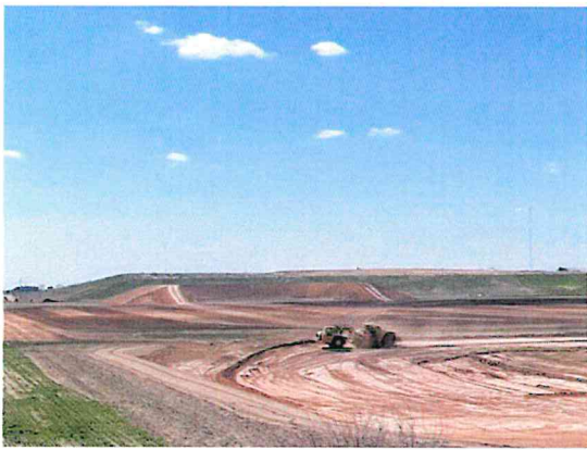
Scrapers hauling dirt to the berm
